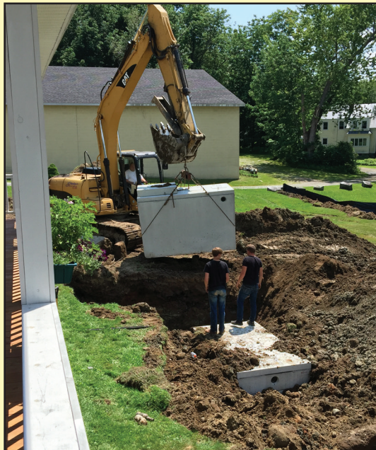
New tank being placed.
