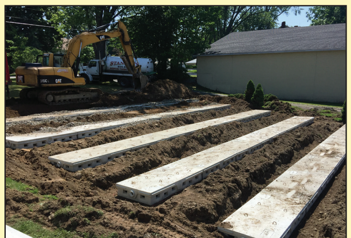
New leach field chambers in place.
